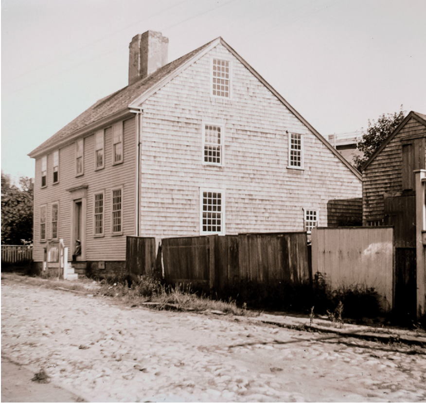
Late-nineteenth-century view of the Macy house on Liberty Street
